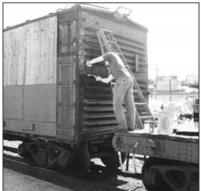
Rome applying rust stabilizer to the A end with view of partly painted plywood.
