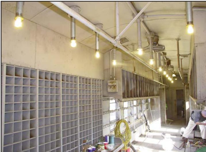
The RPO with lighting. The motion detector switch will save energy by turning on the lights when needed, and automatically shut off the lights when no one is in the car.
