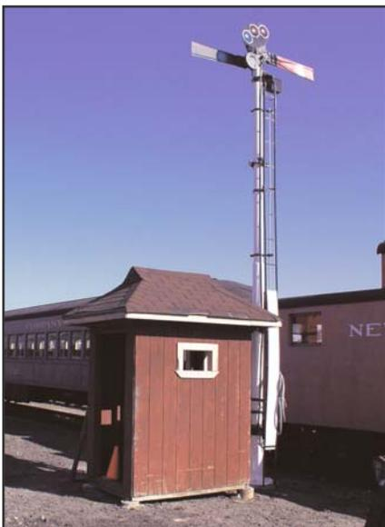
During the past few weeks the Wilton semaphore has been transformed. It now has an operator's shed attached, with the controls to the signal arms positioned within it. Holes were dug for the form cores, which then were filled with concrete as footings. The shed was lifted into place by the trusty backhoe, holes
